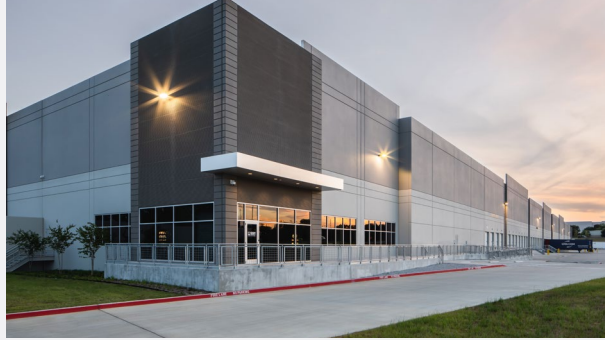
// PARC SOUTHWEST IRVING, TEXAS
