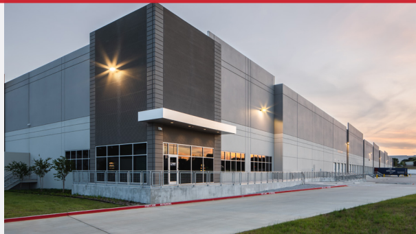
// PARC SOUTHWEST IRVING, TEXAS
