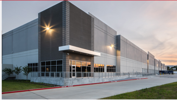
// PARC SOUTHWEST IRVING, TEXAS
