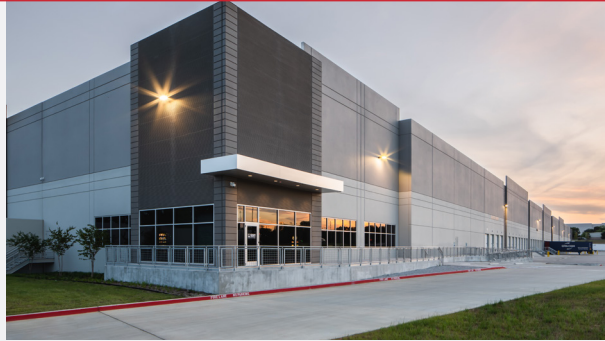
// PARC SOUTHWEST IRVING, TEXAS
