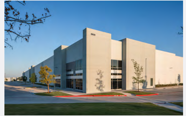
// PARC NORTHEAST RICHARDSON, TEXAS
