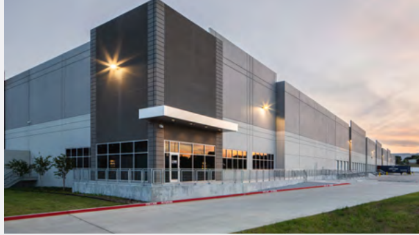
// PARC SOUTHWEST IRVING, TEXAS
