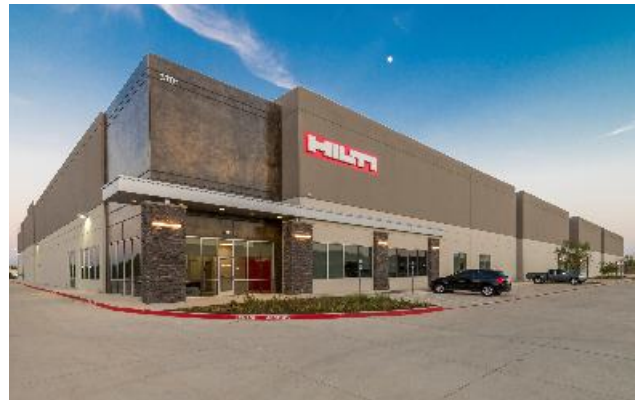
PARC ROYAL Irving, Texas | 5-Buildings | 684,000 SF
