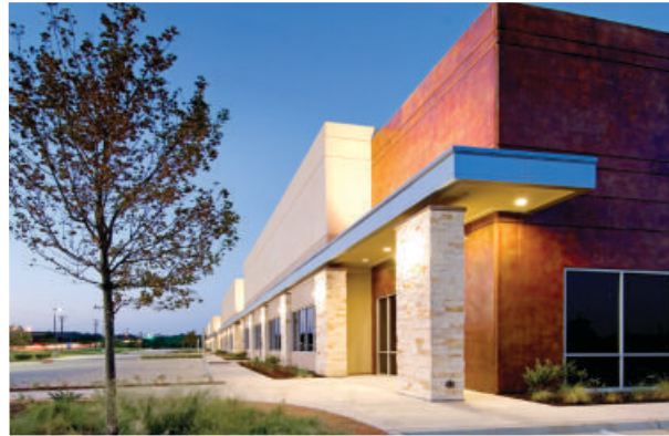
PARC 114 Irving, Texas | 6-Buildings | 406,000 SF
